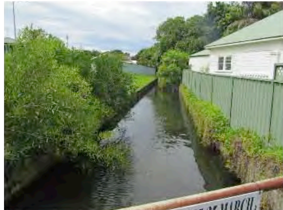
03. View over canal facing East
