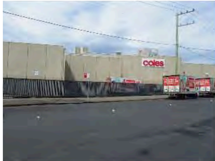
08. Sharp Street facing East Coles loading dock
