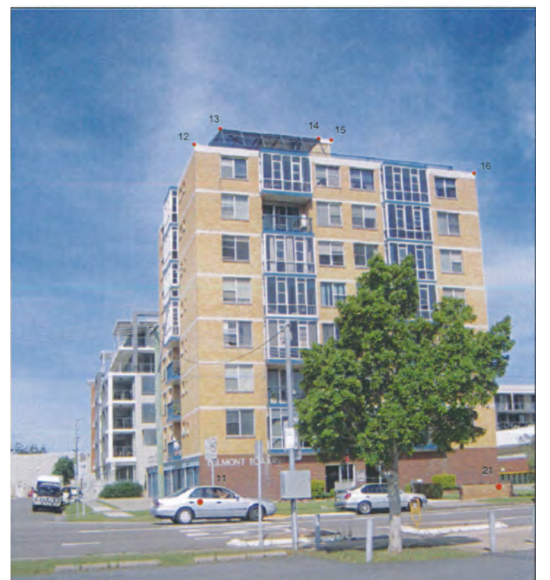
12. Cnr Brooks Parade and Sharp Street facing East Belmont Towers in foreground
